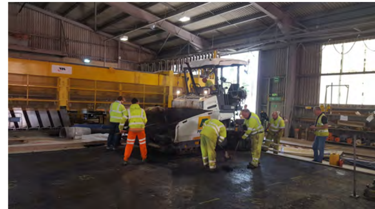
(b) Paving Section 1 base-binder course
