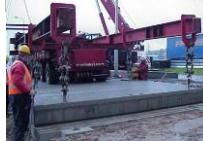
Installation of modular pavement Source: Modi Slab
