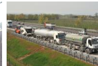
Cold in place recycling on the motorway A4 Turin-Trieste, Italy Source: Wirtgen Company
