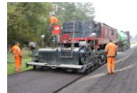
Cold in-place recycling on the state road L 114 in Weilern, Rhineland-Palatinate, Germany Source: Wirtgen Company
